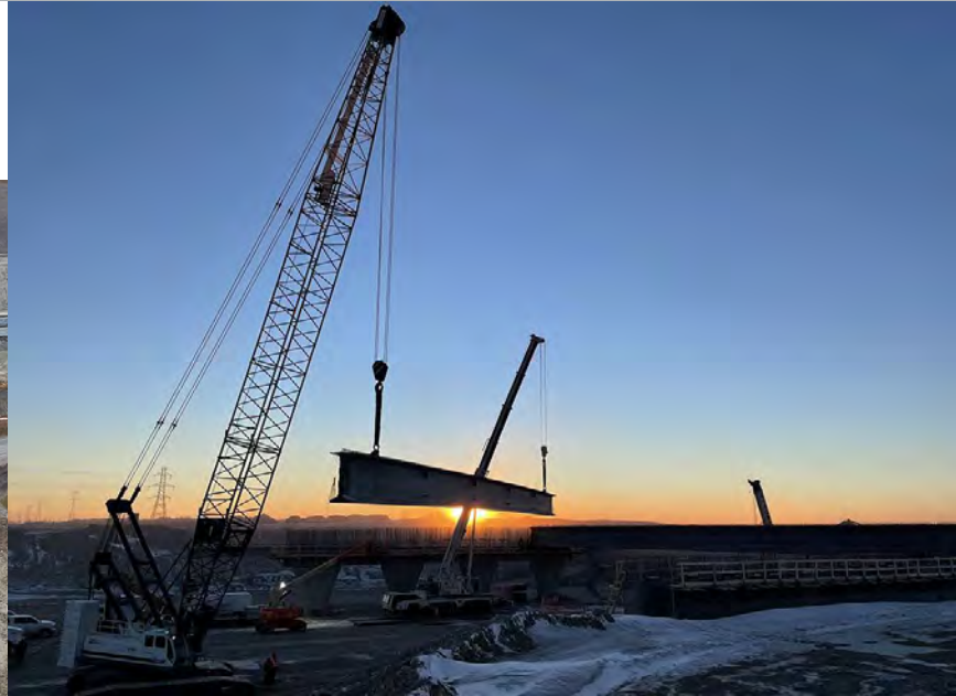
Girder placement at Bow Trail Interchange
