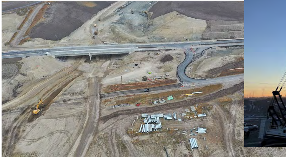
Construction at 17 th Avenue looking north
