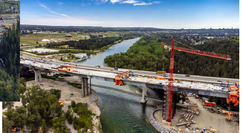
Looking Northeast - Construction Summer 2022
