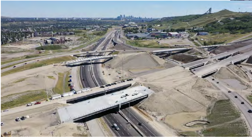
Interchange at Stoney Trail and Highway 1 looking east.
