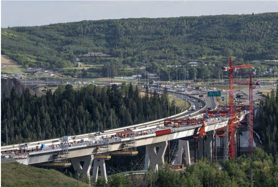
Looking Southwest – Construction Summer 2022
